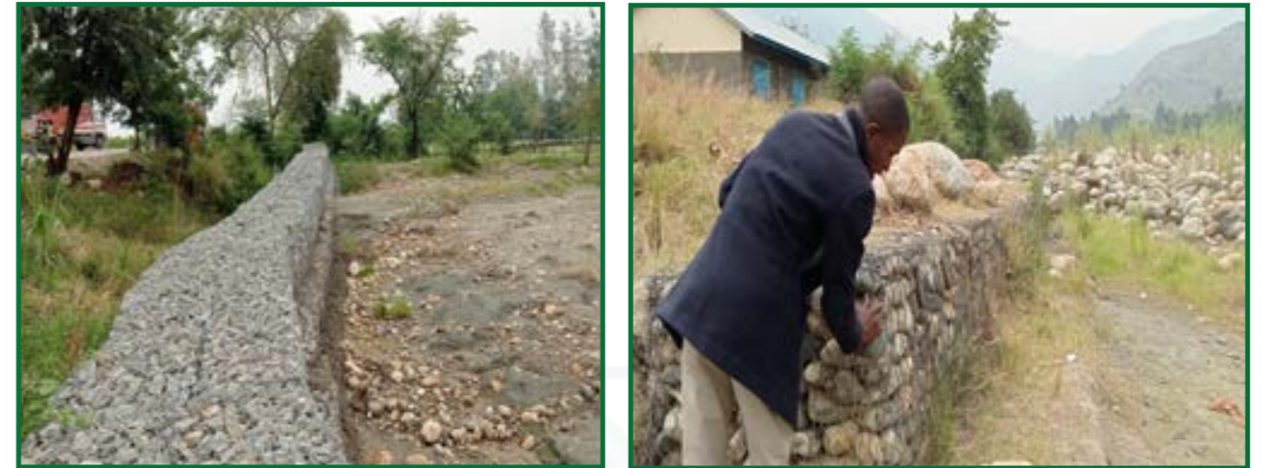
Figure 1: Gabions along some sections of the banks of River Nyamwamba
