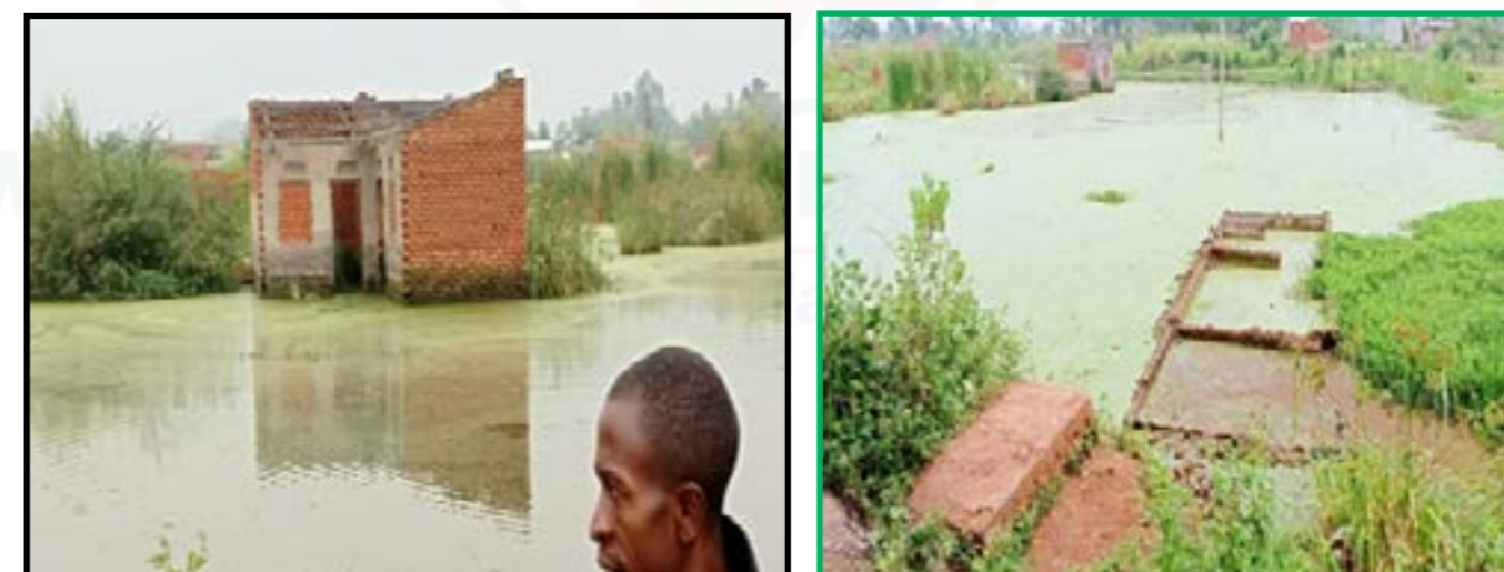
Figure 4: Destroyed households in Kanyangeya Community, Kasese District.
