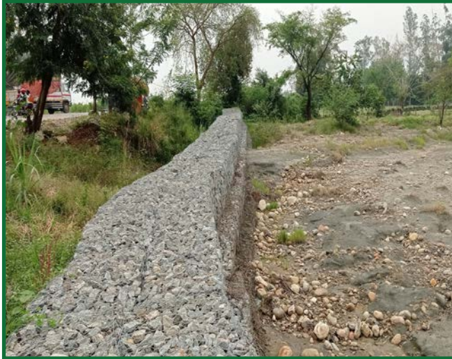
Figure 1: Gabions along some sections of the banks of River Nyamwamba
