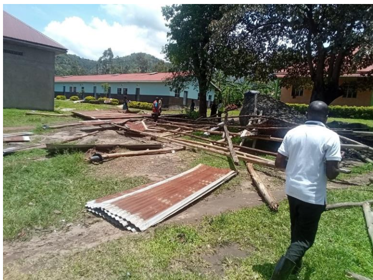
A dining shelter at Mutanywana Sec. School blown off
